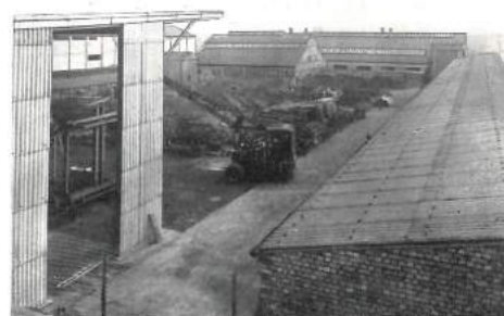
Charlton Works after Extension.
