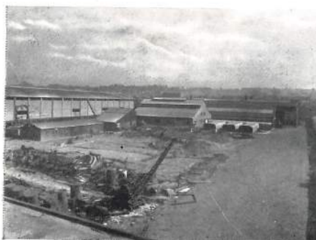
Charlton Works before Extension.
